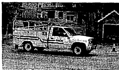
MG&E responded quickly to repair the downed power line.
